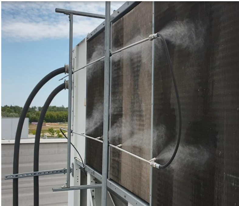
Work completed for two chillers
